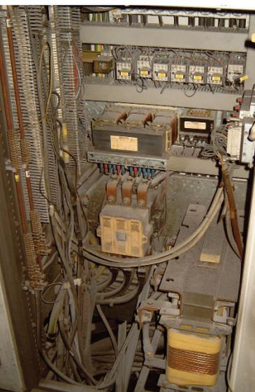
Example of a control panel showing mixed control and power circuits with bare copper busbars
